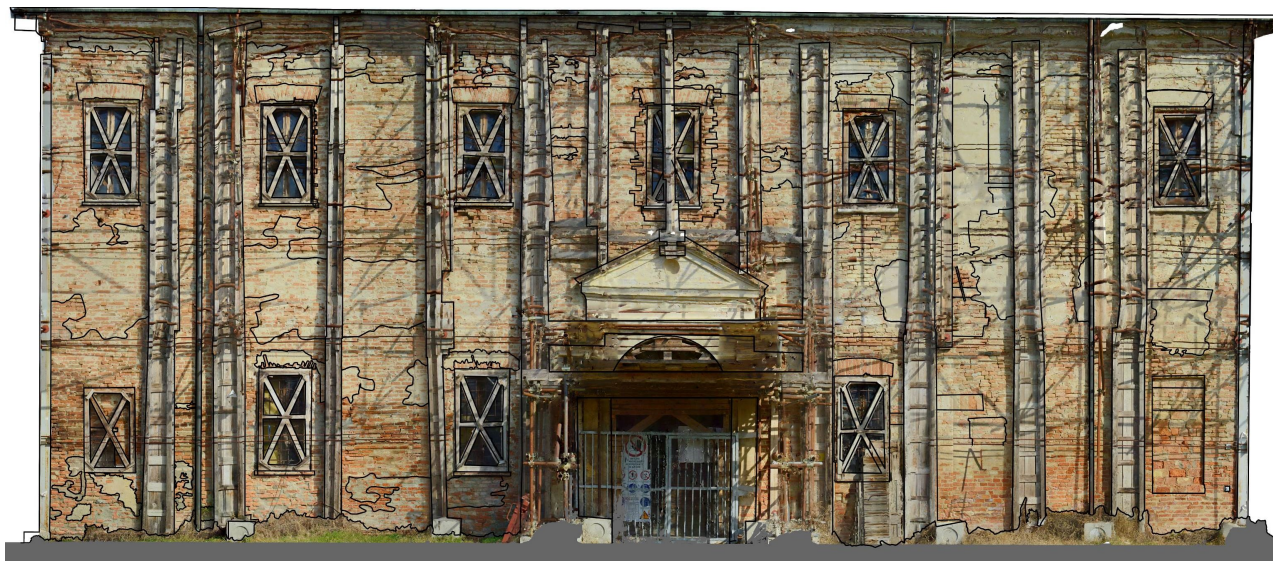
Figure 8: Stratigraphic analysis, first draft. The reinforcement system prevents the correct interpretation of the stratigraphic units.
