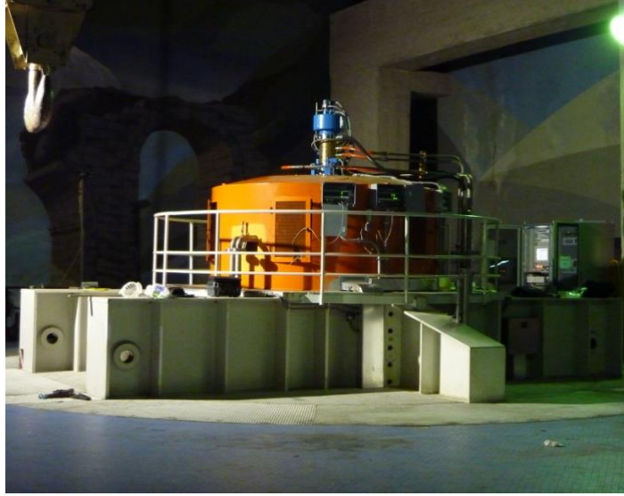
Figure 2. Kaplan turbine unit after installation.
