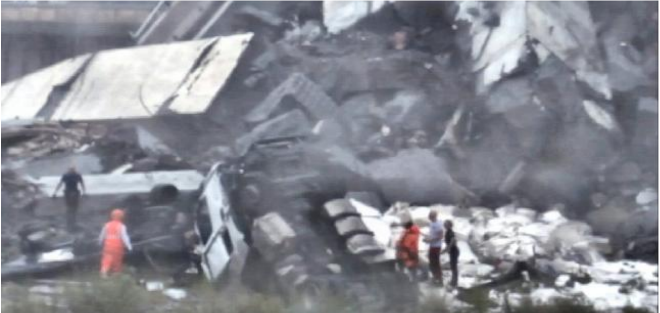
Figure 11. The tractor of the tank between the debris of the bridge.
