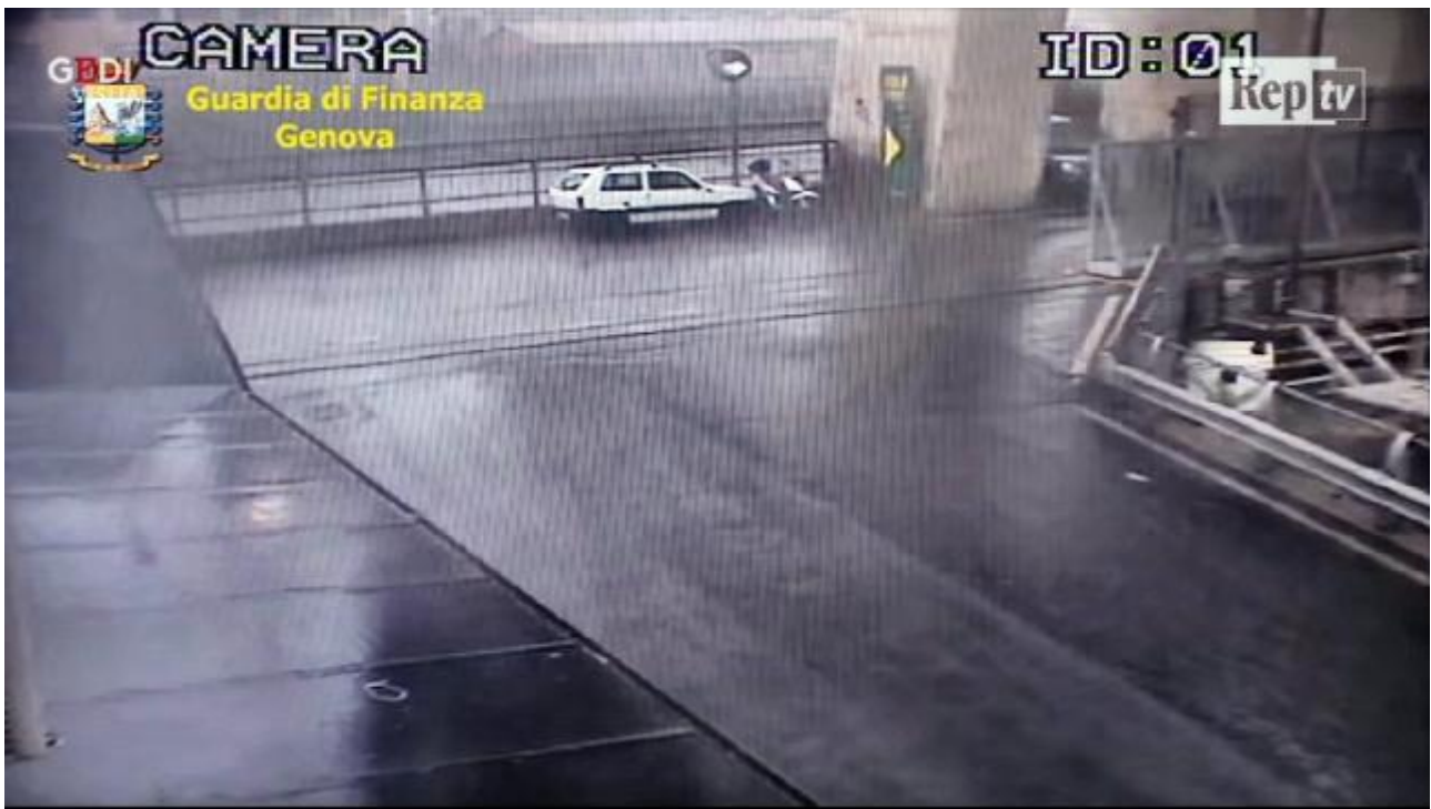
Figure 10 In the webcam under pylon 9, you see a sudden glow: at the top, the reflection of the viaduct on the wet roof. This is a relevant image that helps to determine the speed at which the bridge collapses and the provenance of the debris. This image explains the early phases of the collapse
