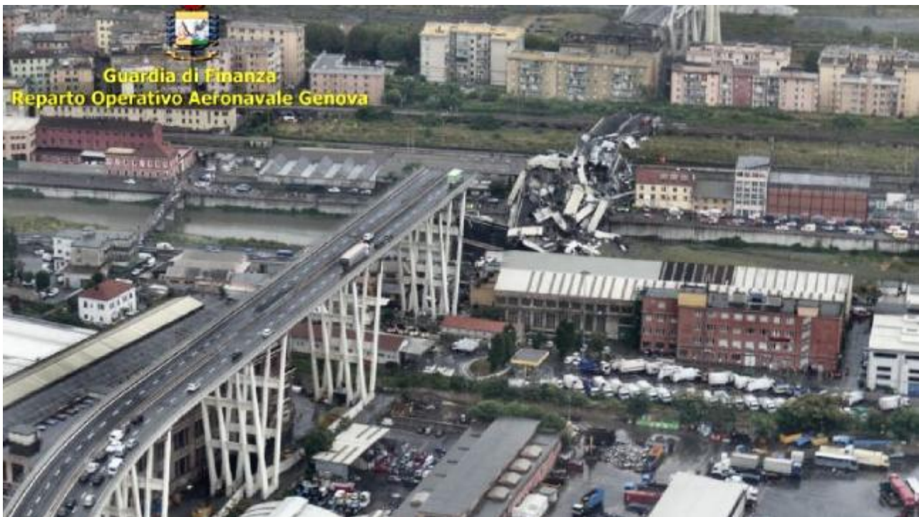
Figure 1 The collapse of the Morandi viaduct in Genoa on the photo taken by the Guardia di Finanza helicopter
