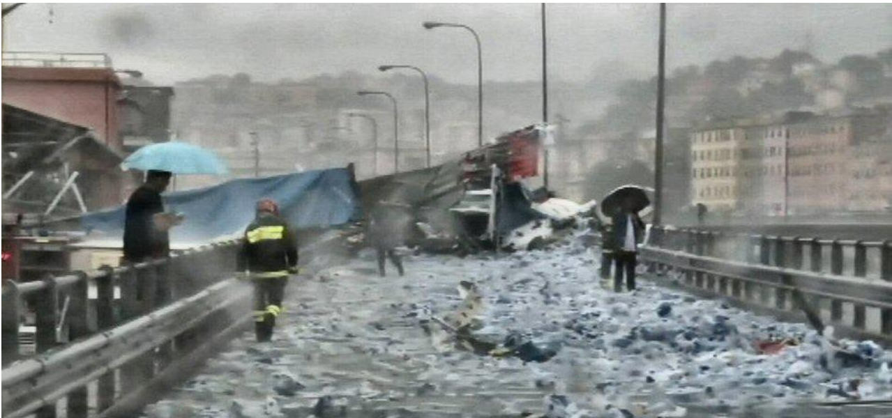
Figure 6 Firefighters run on a surface covered with gravel and small rubble in the whole area of the Polcevera viaduct, Cornigliano side
