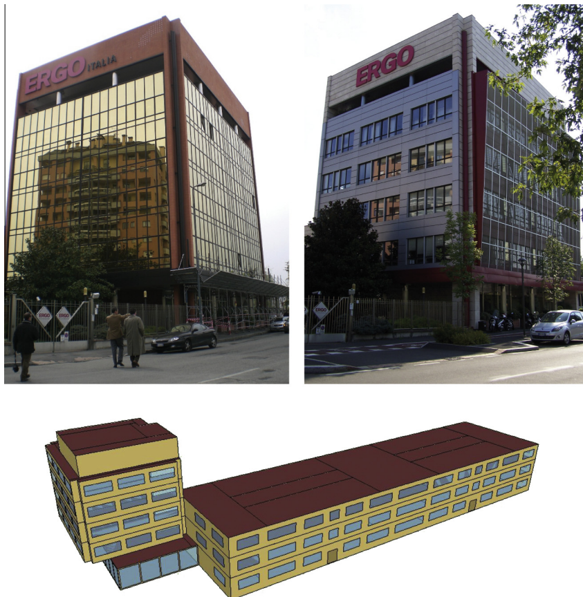
Fig. 2. Real building prior and after refurbishment and building energy model.
