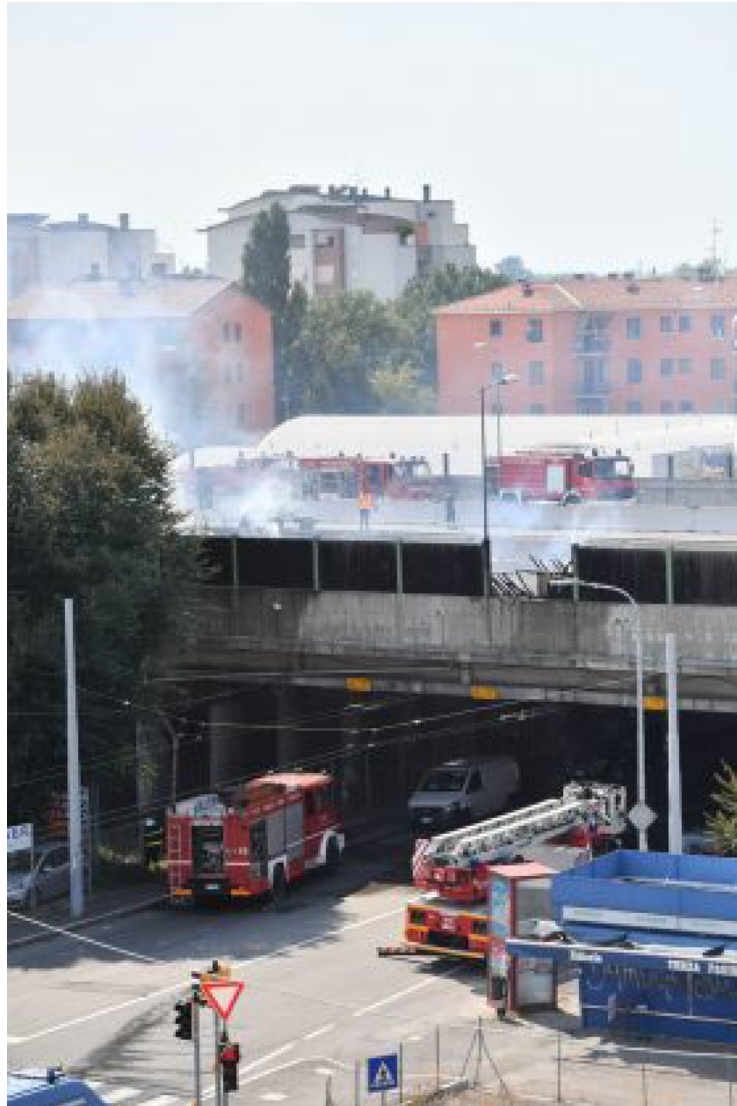
Figure 13 The power cables of the filament line, cables with 600 V voltage, will have been affected by the fire and this led to the explosion.
