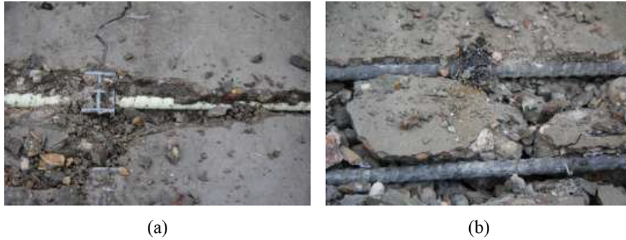
Fig. 17. Post-heating bending. Some rebars after failure of the panels with 5 cm concrete cover. External surface of: (a) Schöck ComBAR® and (b) FiReP® Rebar P.
