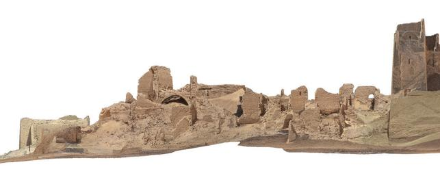
and keeping them structurally sound and stable. In the desert, considering the logistic and environmental conditions, the most efficient system to obtain long-lasting results is to restore the buildings to their original closed shape by using local materials and building techniques. These interventions, however, must be carefully calibrated and tailored to the specific needs of each archaeological site.
