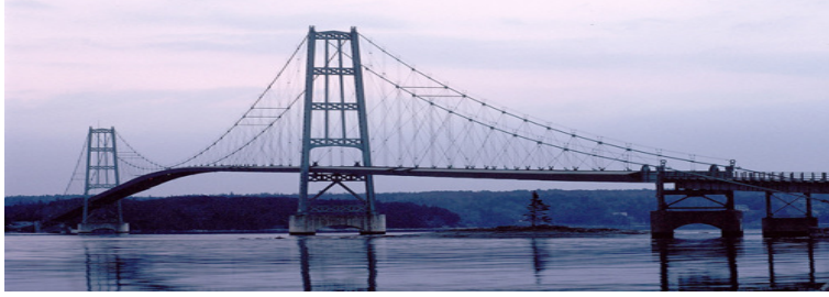
FIGURE 2. The Deer Isle Bridge.
