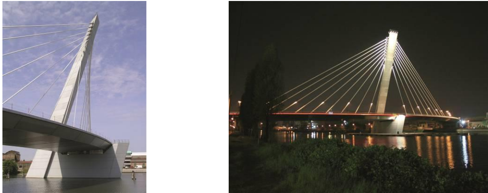
Fig. 9 Views of the cable-stayed bridge in Porto Marghera (Venice, Italy)
