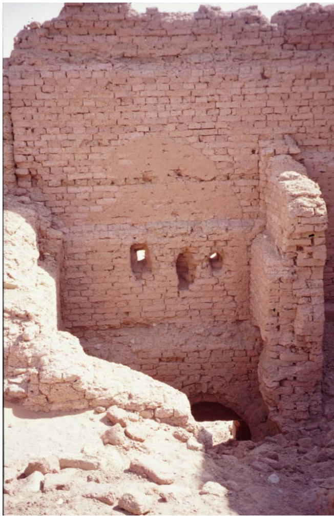
Figure 5: Photograph of the interior of Qasr al-Lebekha (the area of the entrance looking eastwards) showing vertical walls endowed with lateral steps on which the vaults used to rest. Photograph by C. Rossi, 2013.
