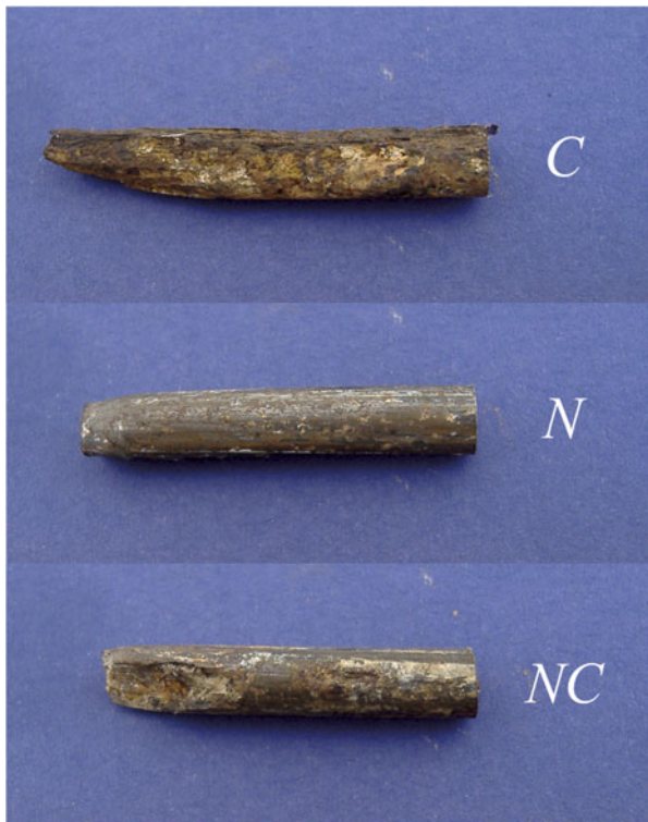
Figure 3. Examples of the types of failure observed on the wires of the tendon failed in service.
