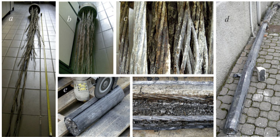
Figure 1. Portions of the failed tendon analysed in the laboratory.
