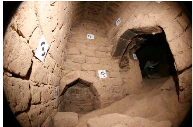
Fig. 3. Targets distributed on the surface of the spaces to be surveyed by fisheye lenses (photograph by F. Fassi, 2015).
