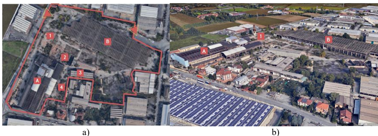
Figure 3. a) top and b) isometric views of the site with access points and main industrial structures.
