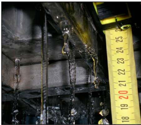
Figure 32. Stainless steel support for the industrial distributors.
