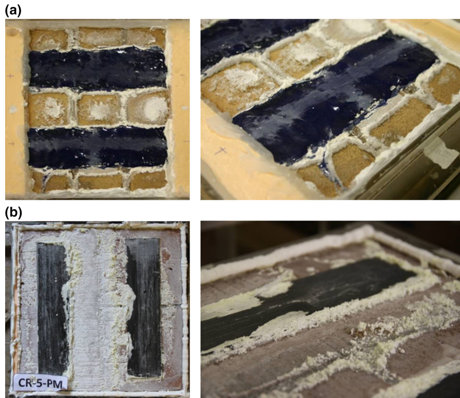
Fig. 7 Damage after 11 cycles of crystallization: a general view and detail of concentration of stresses underneath the fibres in Italian specimens, and b general view and detail of concentration of stresses underneath the fibres in Polish specimens
