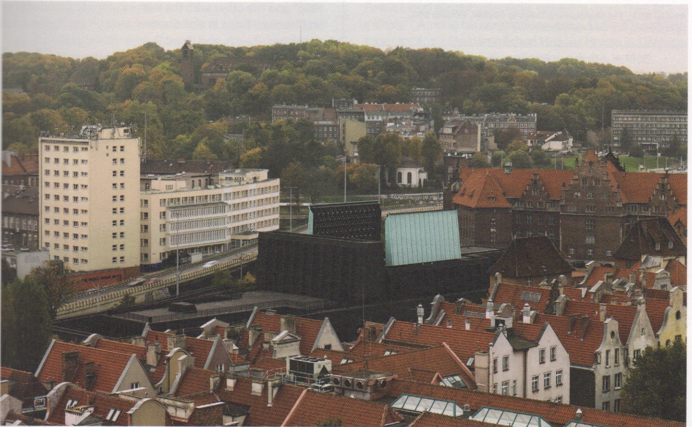
Renato Rizzi, The Shakespeare Theatre, Gdańsk, Poland, 2014. Aerial view of the theater with the roof wings open.
