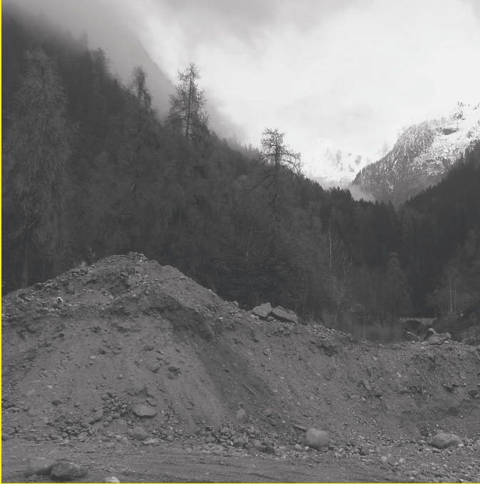
FIGURE 1: Earthwork in the building site (photo Chiara Pradel).
