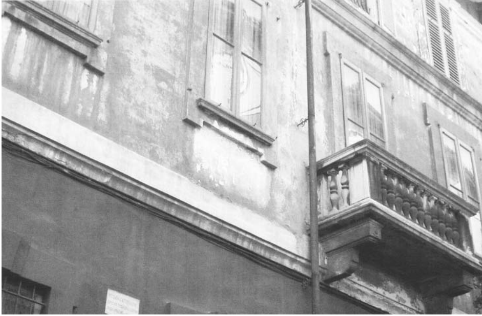
FIGURE 8 A house in Milan with secondary glazing.
