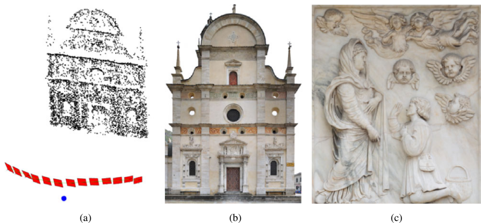
FIG. 3. The main façade of the Sanctuary of Tirano, Valtellina, Italy. (a) The result of the combined orientation of central perspective images (red squares) and one gnomonic projection (blue circle): black dots are the 3D coordinates of tie points on the building façade. (b) The entire rectified projection (1 pixel = 1 mm) generated from the integrated approach. (c) Detail from the rectified projection.
