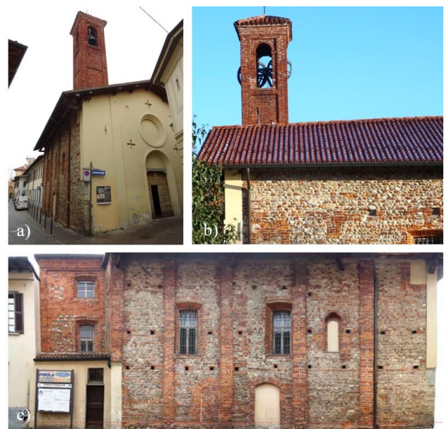
Figure 2. St. Antonio Oratory: a) the façade; b) the bell tower and c) the rectified north side with its stratifications.
