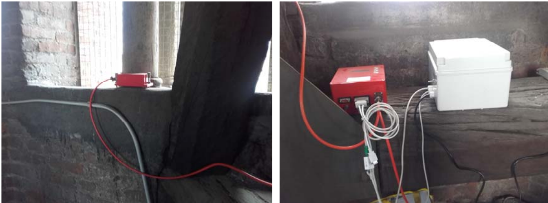
Figure 3: Measurement devices installed in the San Gottardo bell-tower.
