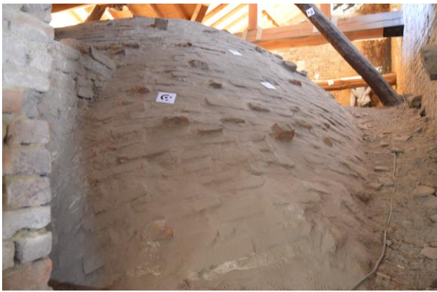
Figure 2. Magio Grasselli Palace: extrados of the staircase vault (Room 1.26).
