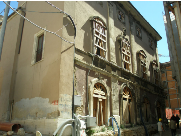
Figure 2: Masonry façade object of the study.
