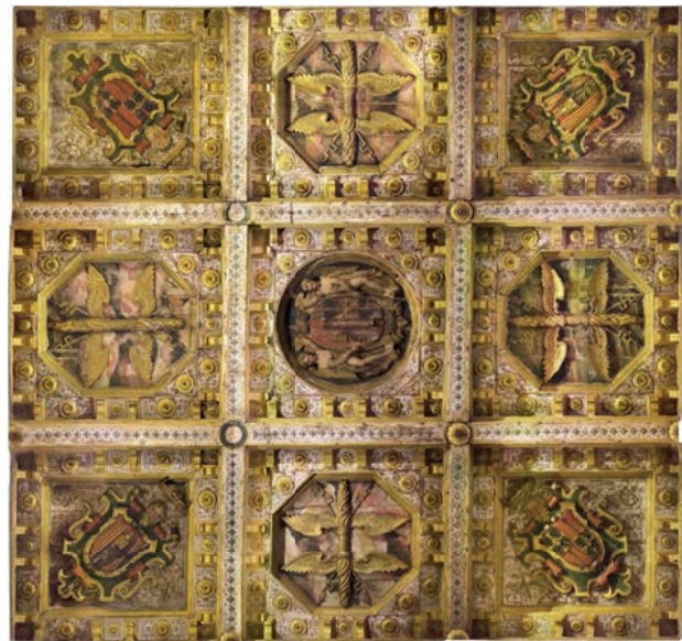
Figure 9. Details of the ceiling coming from Photoscan projections
