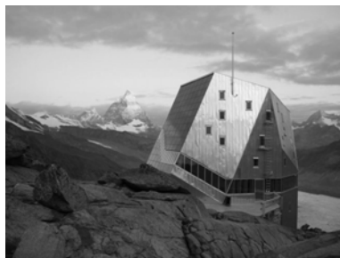
Rifugio sul Monte Rosa, Bearth & Deplazes, 2009 (fonte: https://www.archdaily.com/802453/monte-rosa-hut-bearth-and-deplazes-architekten )
