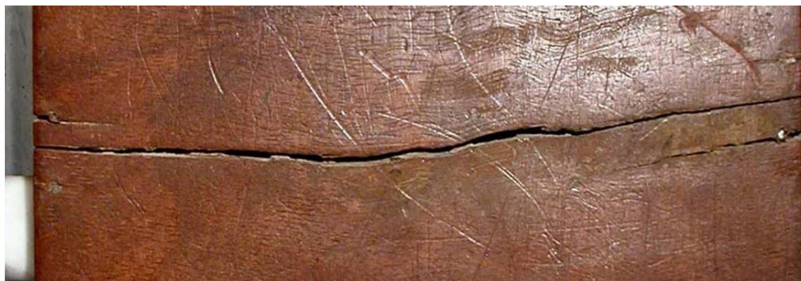
Figure 11. Detail of the outer side of the bottom. Irregular fissures—some of them favored by the insertions of “modern” nails.
