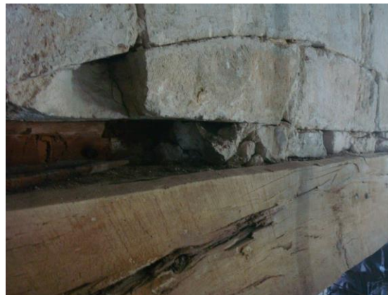
Figure 18: Filling material between relieving arch and lintel.
