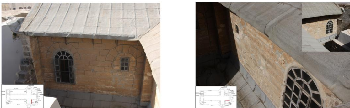
Figure 5: Walls of the corners.
