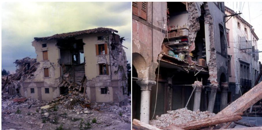
Fig. 5 - Damage in the Friuli 1976 earthquake.
