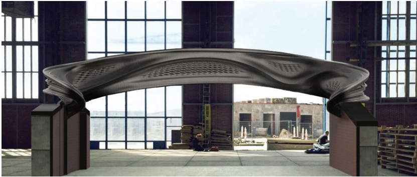
Figure 13. Robotically printed metal bridge ( https://tinyurl.com/yanqvhv9 ).
