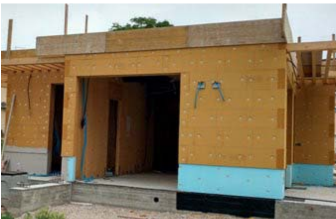
05-06 | Demonstrator building, Benevento. Construction phases: assembly of X-Lam panels (Cross Laminated Timber) and stratification of the external walls. The choice of the Fibertherm Flex 180 panel contributes to ensure a good thermal inertia thanks to its mass, making it suitable for the reference climate context
