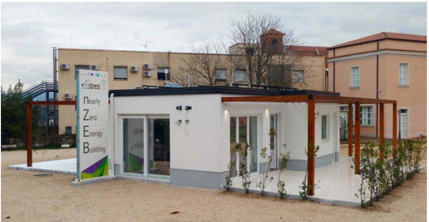
07 | Demonstrator building, Benevento. nZEB near completion
