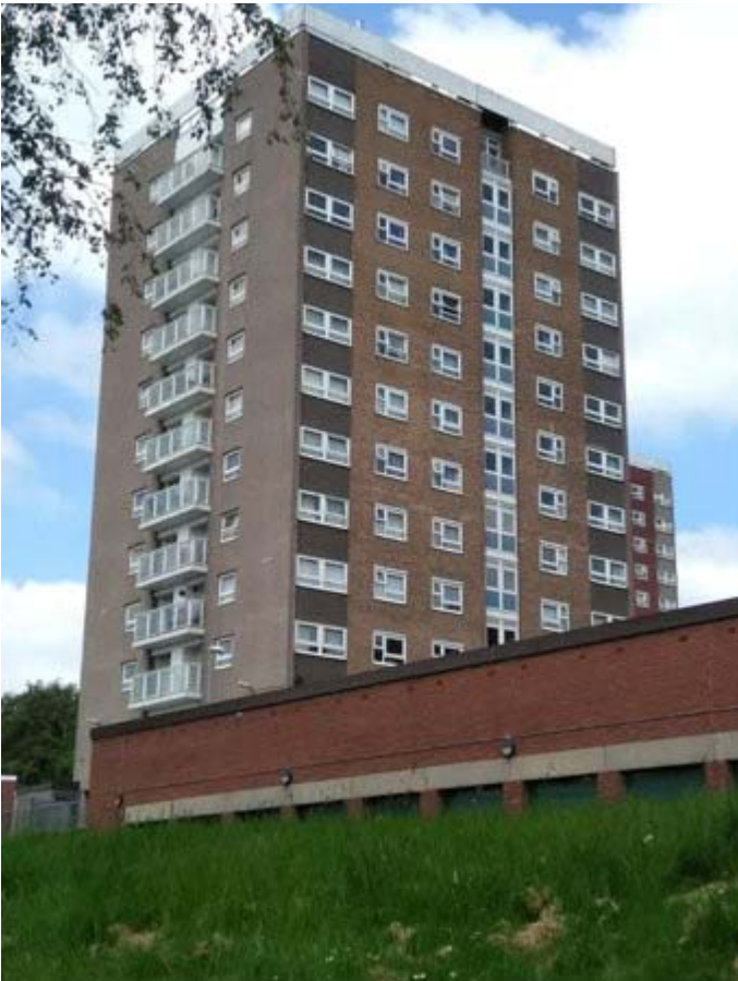
02 | Leeds tower blocks in their current conditions (Photo: O. Iuorio)
