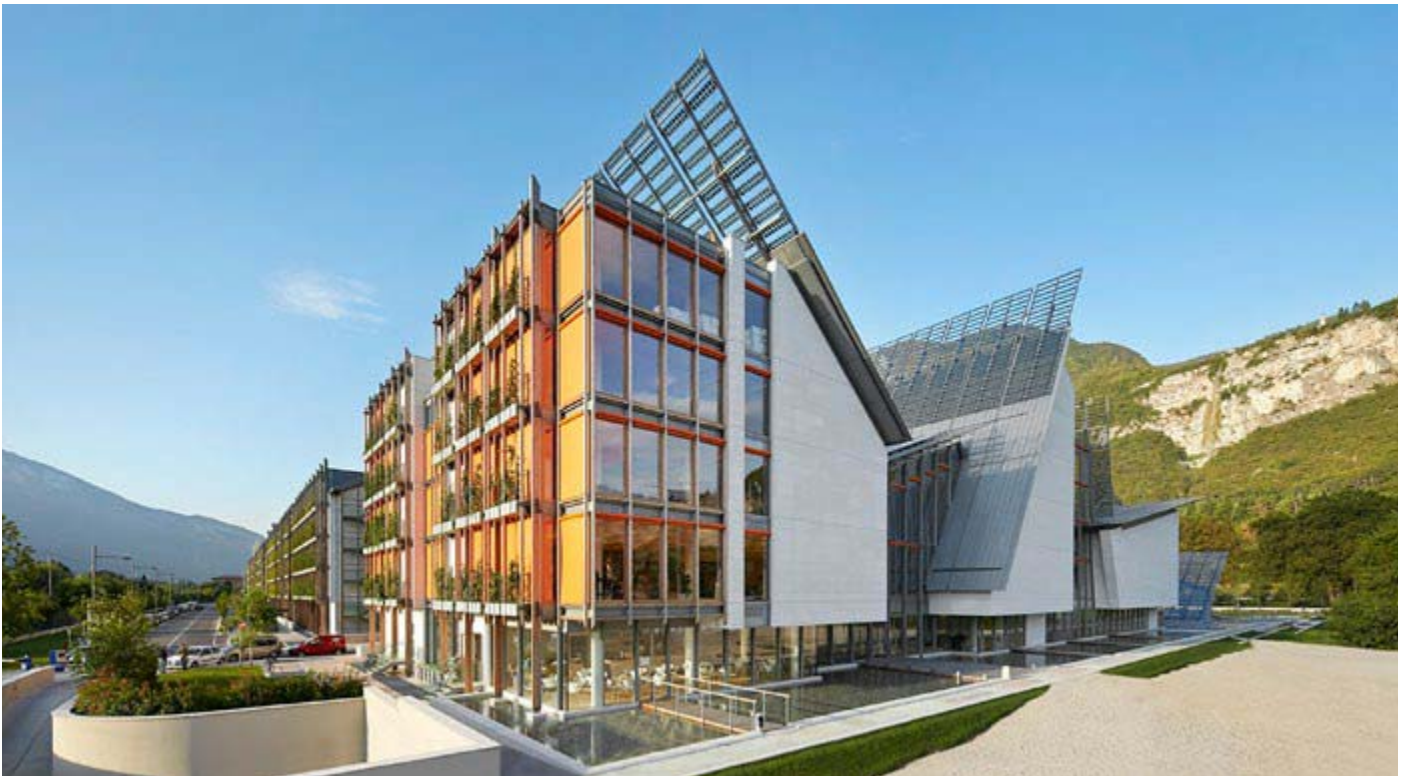
02 | The Gold LEED certified Sciences Museum "MuSe" (RPBW, 2002-2013) is located in the post-industrial brownfield of "Le Albere", thus reinforcing the cultural identity of this area of Trento. Image credits: Hufton+Crow
