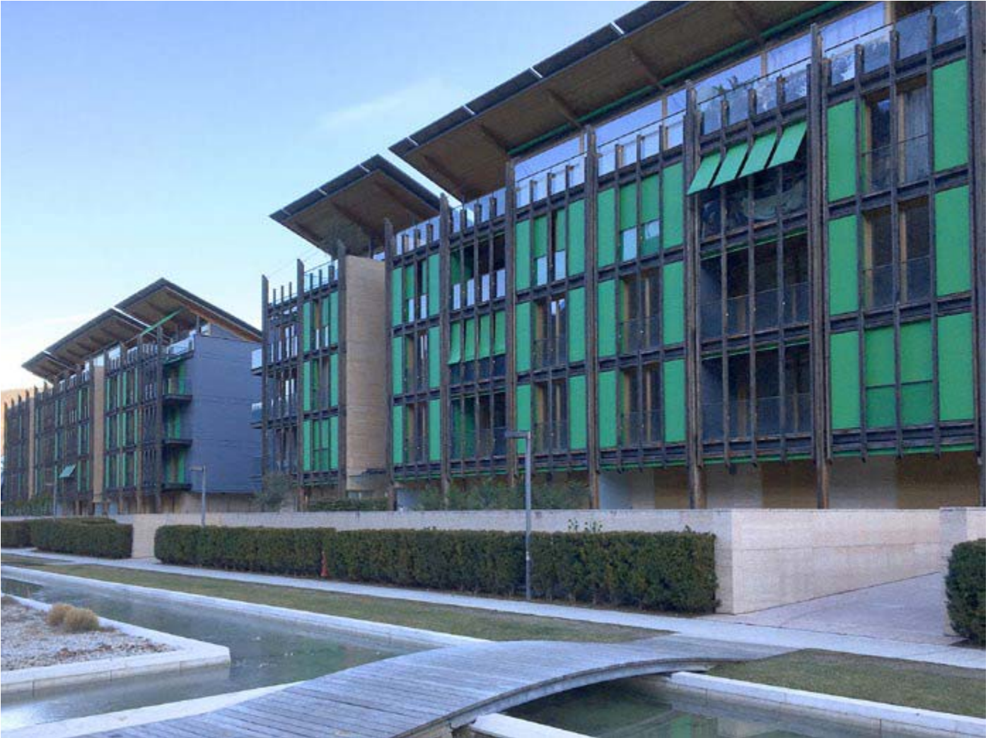
01 | "Le Albere" green neighborhood (RPBW, 2002-2016), 11 hectares urban expansion in a former Michelin factory site in south-west Trento. Image credits: M. B. Andreucci
