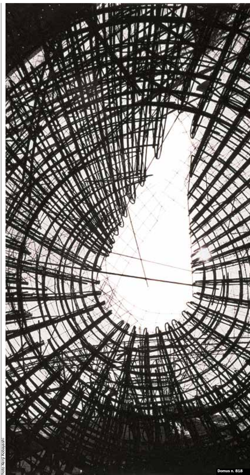
1999 L'armatura metallica della Truss Wall House di Ushida Findlay Architects a Tokyo/ Metal reinforcement of the Truss Wall House in Tokyo by Ishida Findlay Architects
