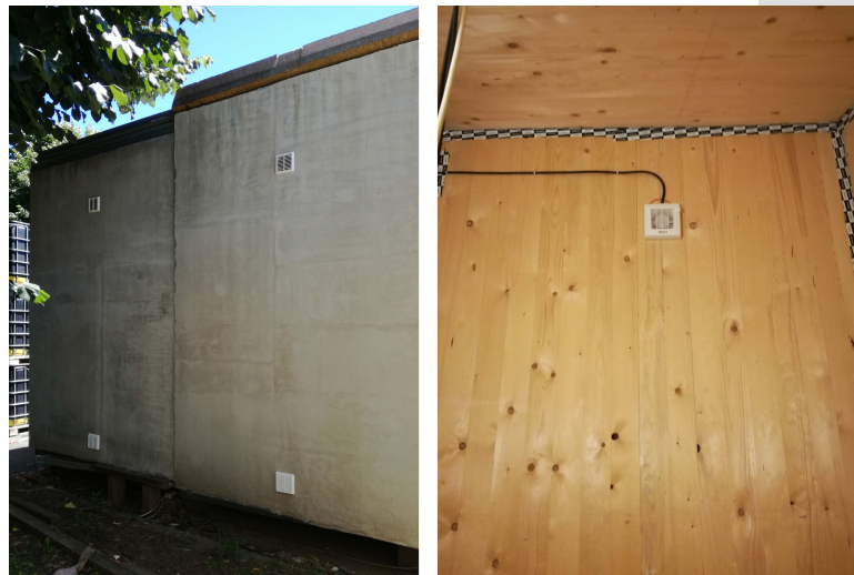
Figure 9. North façade of the test box. The white elements on the façade represent the ventilation extract fans and the ventilation grilles. The Test 3 was set to analyze the night ventilation effect on the two analyzed envelope technologies.
