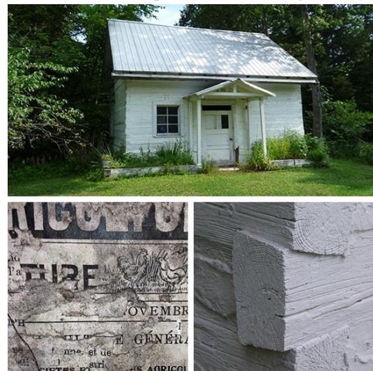
Figure 1. Breard Log House – Newspaper (1899) – Cornerwork (dovetail)
