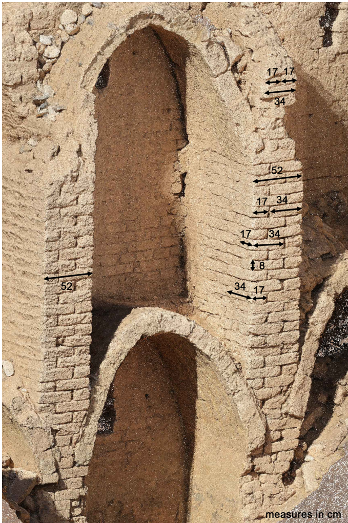
Fig. 7 Axonometric view of a detail of the point cloud (along the interior of the northern side of the Fort) showing the mudbrick pattern and its dimensions (cf. Fig. 2 for the position of this wall)
