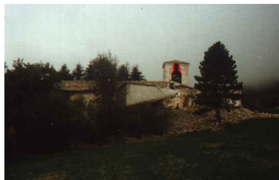
Figure 12. The image shows the state of damage post the 1997 earthquake of the east side of the building. In the foreground, the portion of the collapsed monastic complex is visible, while in the background, the damaged bell tower appears [56].
