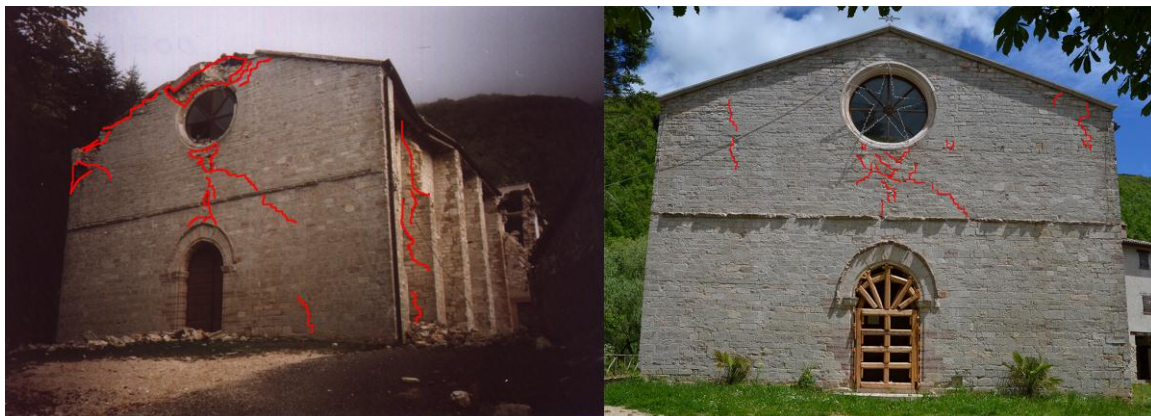
Figure 21. Comparison of the state of damage on the façade after the 1997 earthquake (on the left) and the 2016 one (on the right).
