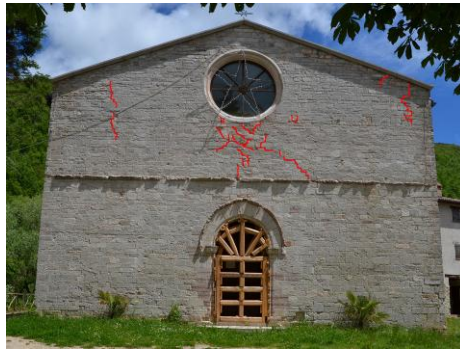
Figure 18. Post-2016 earthquake damage of the external façade with the damage pattern.
