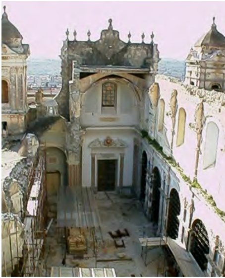
Fig. 15 View of entrance of Noto cathedral after removal of ruins
