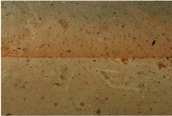
Fig. 18 Couple of bricks with original joint
