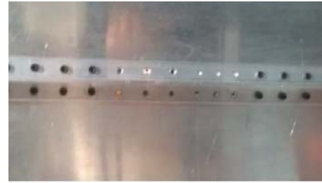
FIGURE 6: Detail of D3 damage.
