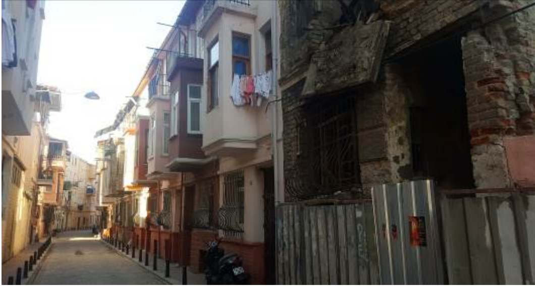
Fig. 3 - 19 th century row housings and urban pattern, personal archive, photo by Emre Kishalı.
