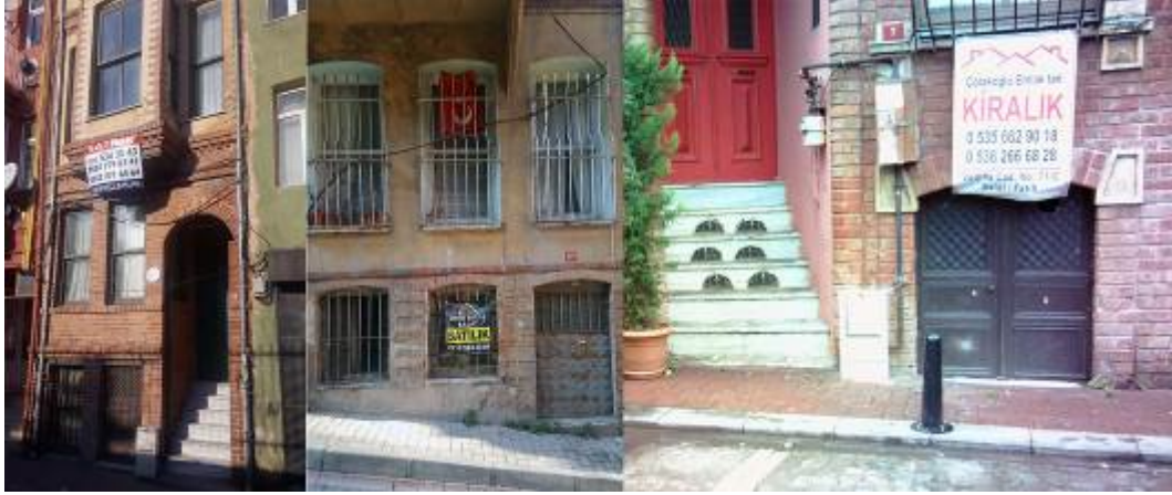
Fig. 7 - Rehabilitated buildings on sale and for rent in 2017, personal archive, photos by Emre Kishali.
