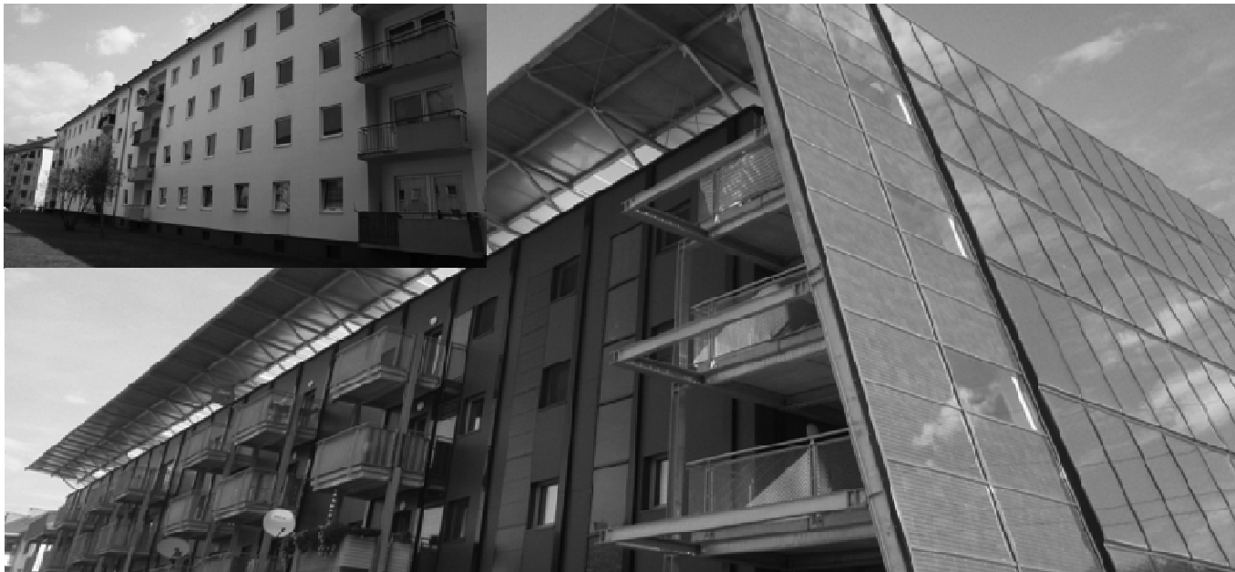
View of existing (small picture) and the renovated building (large picture) (west elevation)
