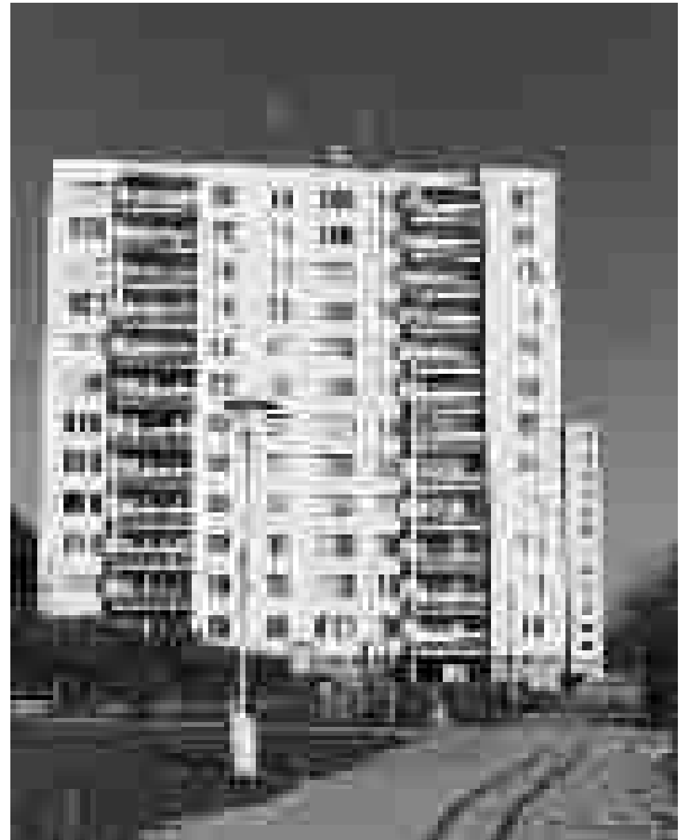
Western view of renovated Koniklecová 4 block-of flats.
