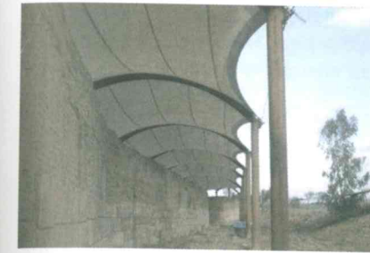
Figure 1. Covering system in Caposoprano, Gela (Sicily). Picture by Canobbio.
