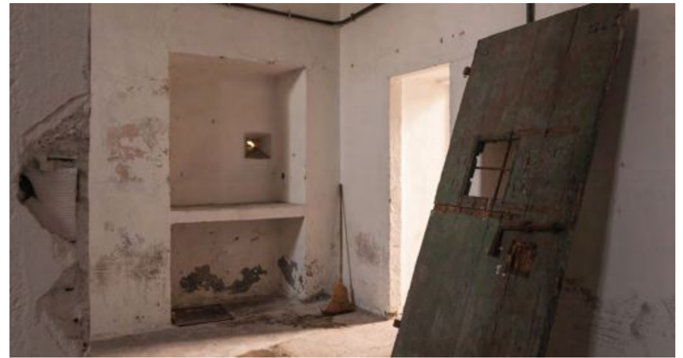
Santa Agata Former prison. View of the former prison cells hosting the exhibition "Envisioning Santa Agata" (October 2017), featuring works by MA students of the Architectural Preservation Design Studio (a.y. 2016-2017), School AIUC - Politecnico di Milano (Professors Fernando Vegas Lopez-Manzanares, Francesca Lanz and Rajendra Singh Adhikari). © Giovanni Galanello
