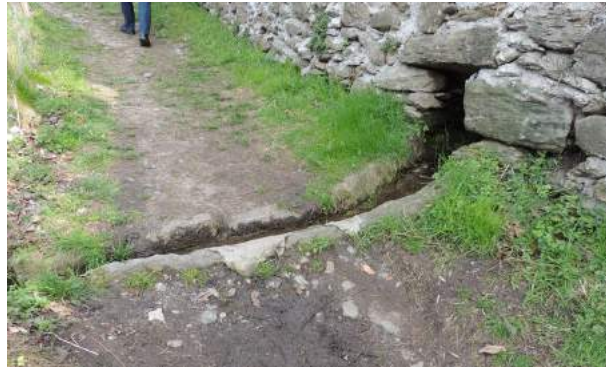
Fig. 4 - Ancient canalisation help the draining system of the drystone wall. (photo: Andrea L'Erario)
