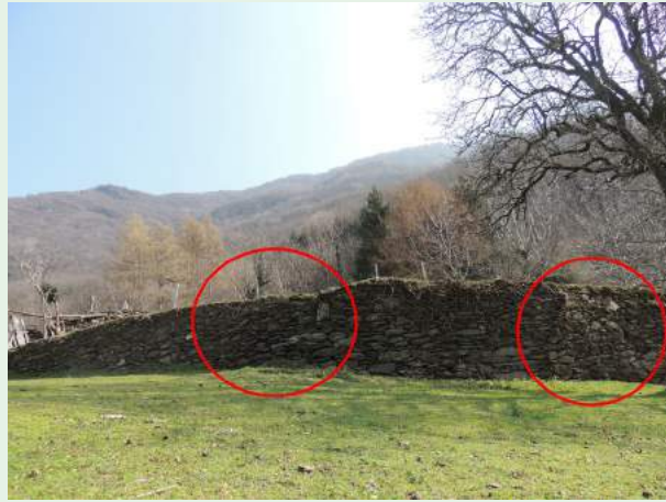
Fig. 30 - Two level junctions in the wall are visible in the red circle. (photo: Andrea L'Erario)
