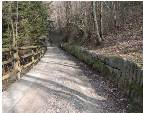
Fig. 6 - The Viandante pathway in the south part from Mondonico to Dervio does not conserve historical characteristics: dimensions have been changed for being vehicle accessible and historical elements now include concrete reinforcements. The new wood railing is too smooth and its forms belongs to wood industry not handcrafted production. (photo: Andrea L'Erario)
