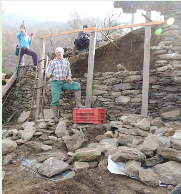
Fig. 31 - Accomplishing the repair of a wall provides great satisfaction! It is proud work! (photo Andrea L'Erario)
