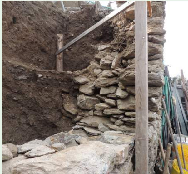
Fig. 28 - Section of a wall under construction: here the horizontal lay out of stones are clearly visible, the vertical alignment helped by a wood post, the difference between the big stones in the front and the small stones for the drainage at the back. (photo: Andrea L'Erario)
