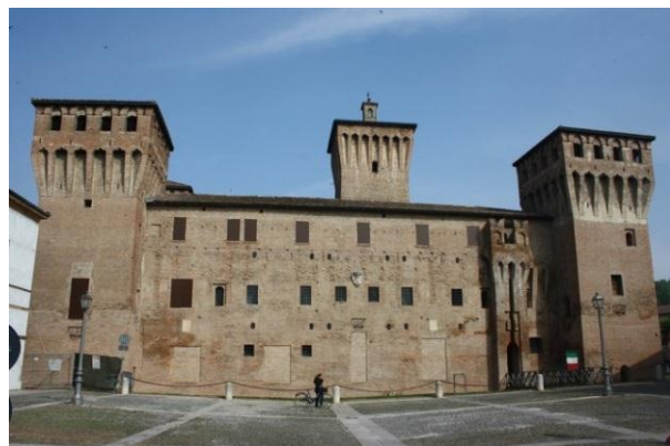
(b) Main façade refurbished
