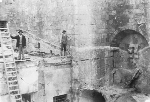
Fig. 13 Prisons demolition. The signs are still visible on the walls
