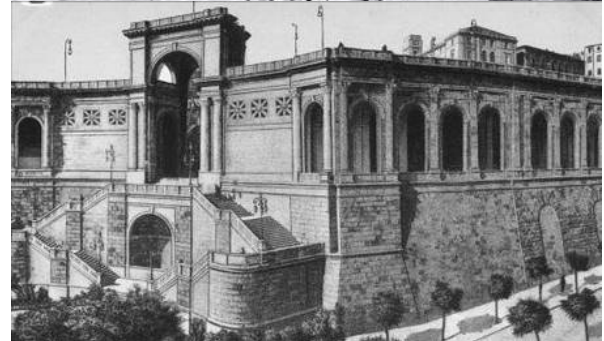
Fig. 6 Cagliari, southern bastions at the end of 19th century: structures built against the walls are clearly visible. They were later removed to build the Bastion of San Remy
