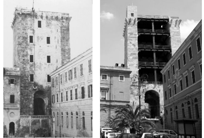
Fig. 14 San Pancrazio Tower before and after the wall demolition
