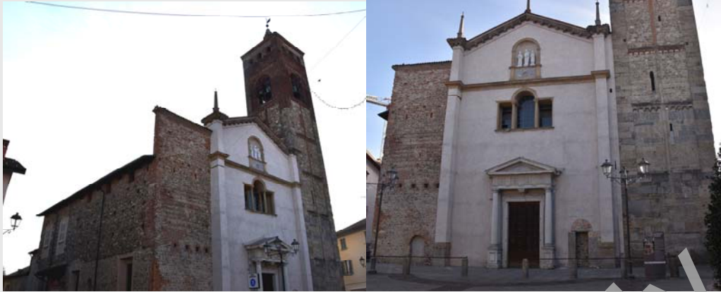
Figure 3: Views of the church of St. Stephen
