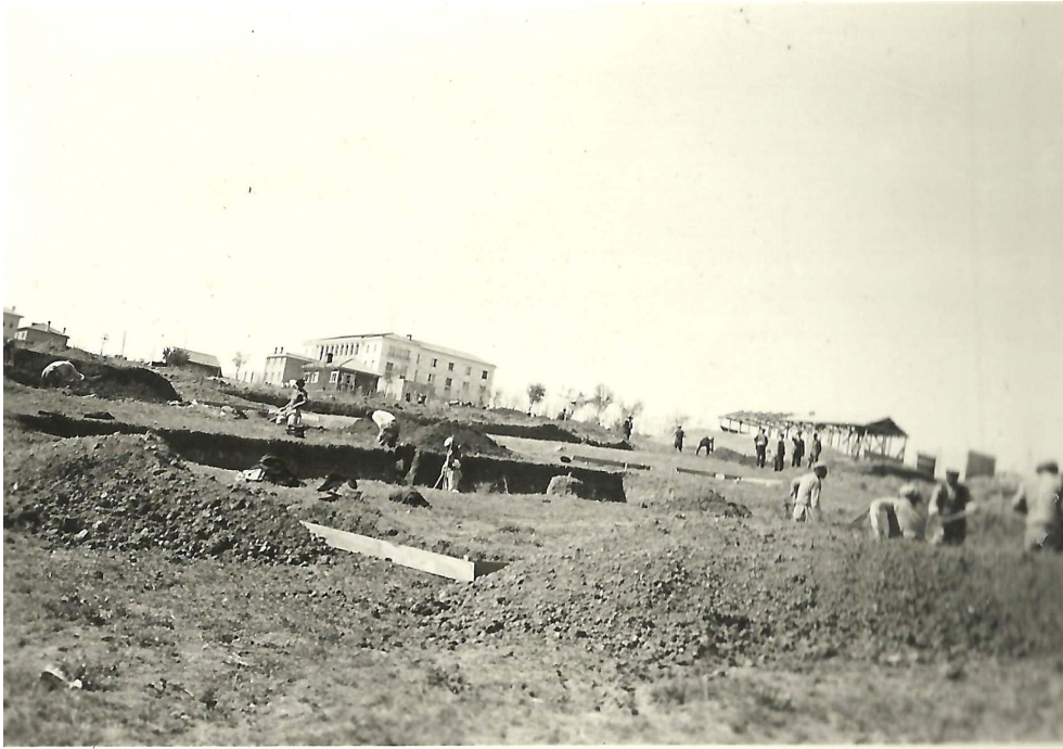
Figure 7: Paolo Caccia Dominioni, excavation works for the church (building A) and the Records' Office (building B).
