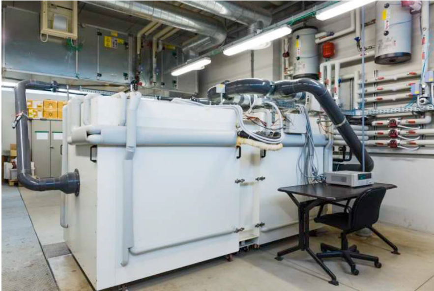
Fig. 3. Picture of the DAVTB facility. The boxes (with the interposed sample frame) are visible, together with the hydronic plant and the air recirculation system.
