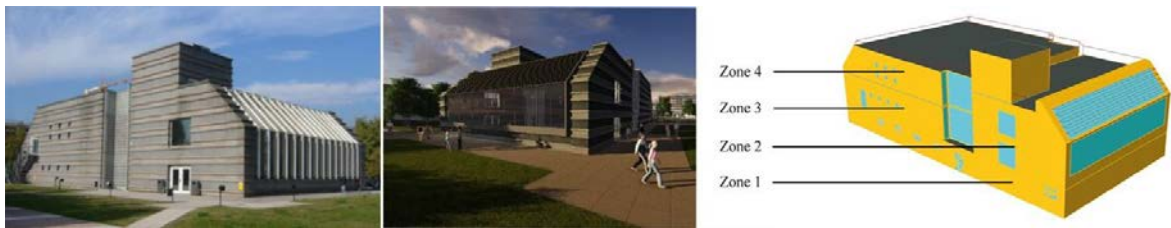
Fig. 3. South-west and south-east façades of the eLux Lab at the University of Brescia Smart Campus, BIM model and BEM with thermal zoning.
