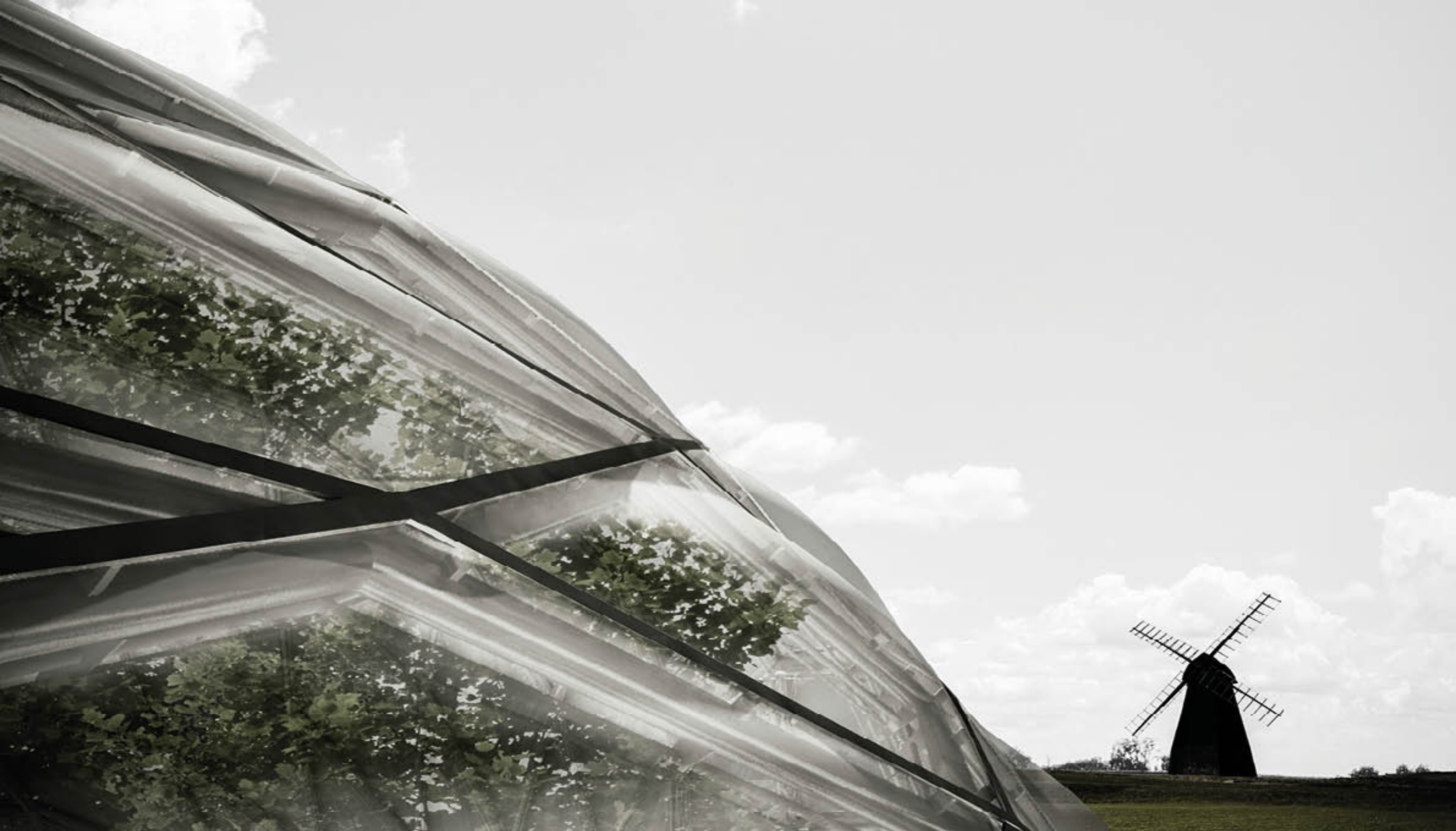
View of roof details
