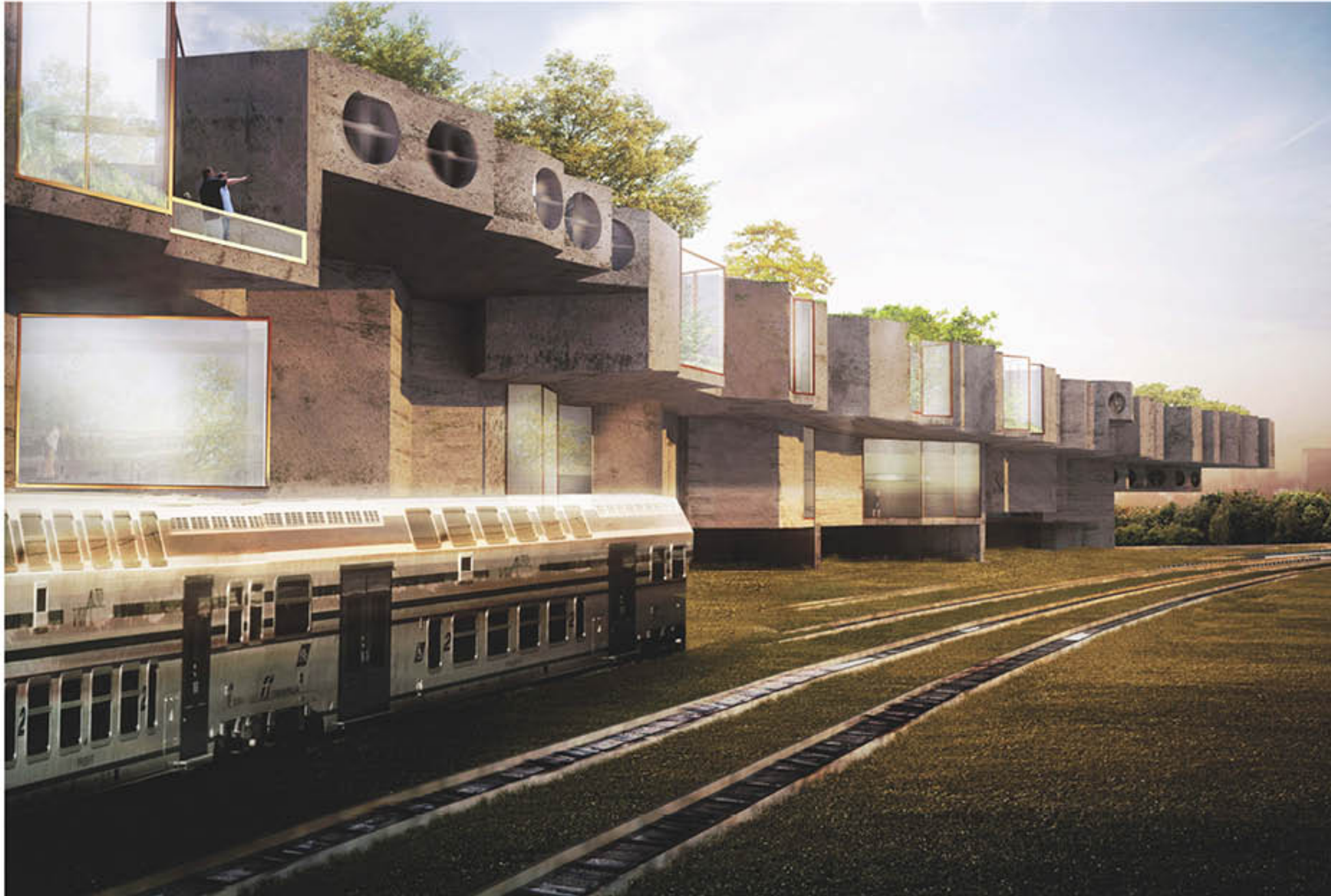
The Zero Energy wall / The new urban wall facing the railroad, with residential units and wind turbines integrated into a compelling new architectural language. The folded geometry of the building's front refracts the noise generated by passing trains, while the innovative cladding material absorbs excessive sound before reaching the building's interior.
