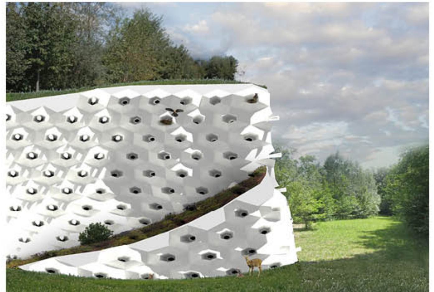
The retaining wall as modular system of cells
