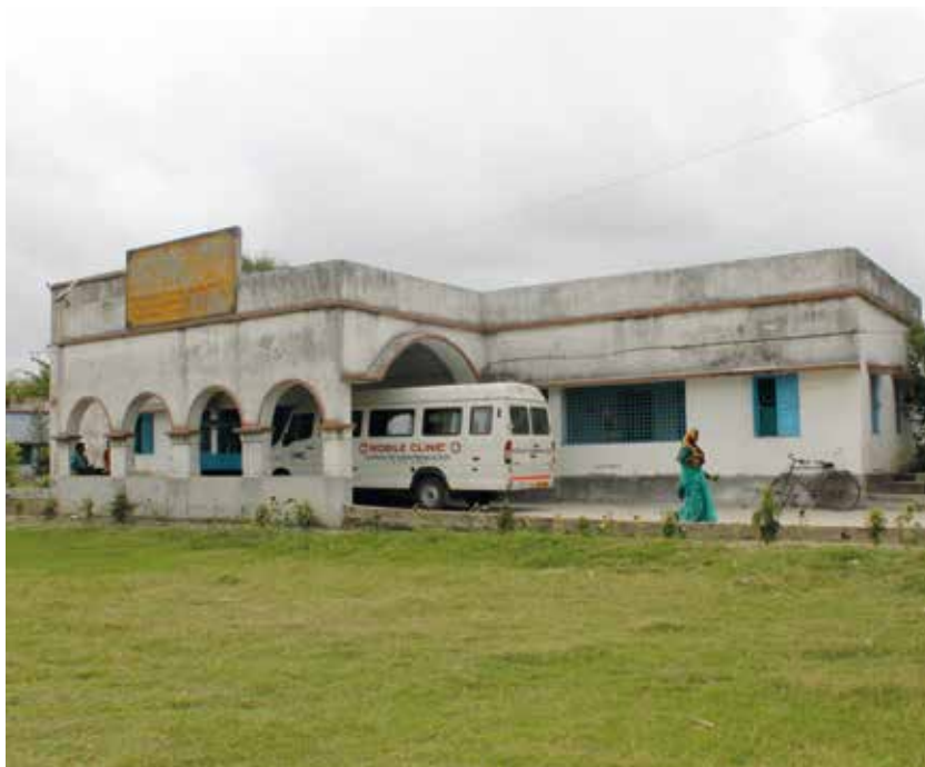
Rilievo fotografico, clinica Dhaki IIMC Photographic survey, Dhaki IIMC Health Centre
